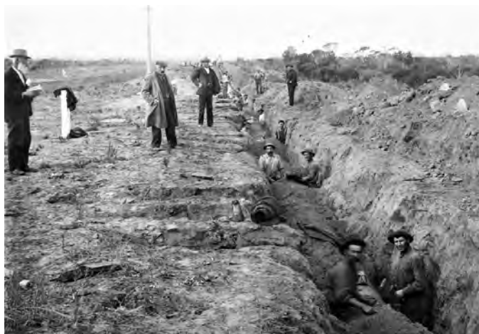
Supervising the laying of the goldfields pipeline near Merredin
