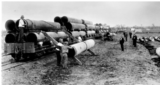
Unloading pipes from a train for the Goldfields Water Supply Scheme
